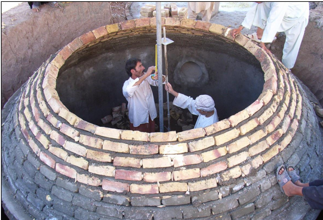
Anaerobic digester under construction in Afghanistan (Credit: SuSanA)
