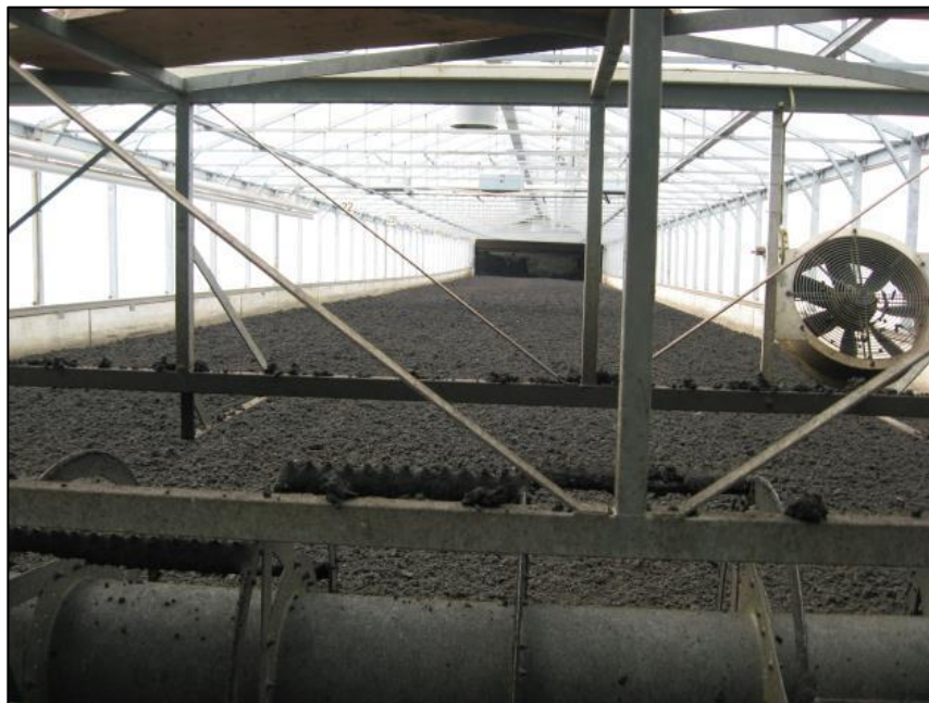
A thermal dryer used for drying wastewater sludge before combustion in Switzerland (Credit: Eawag-Sandec)
