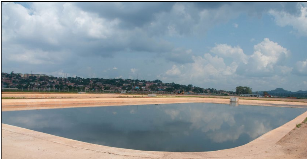
Waste stabilization ponds are a common effluent treatment technology for faecal sludge, here from settling-thickening tanks and drying beds in Kampala, Uganda. (Credit: Eawag-Sandec)
