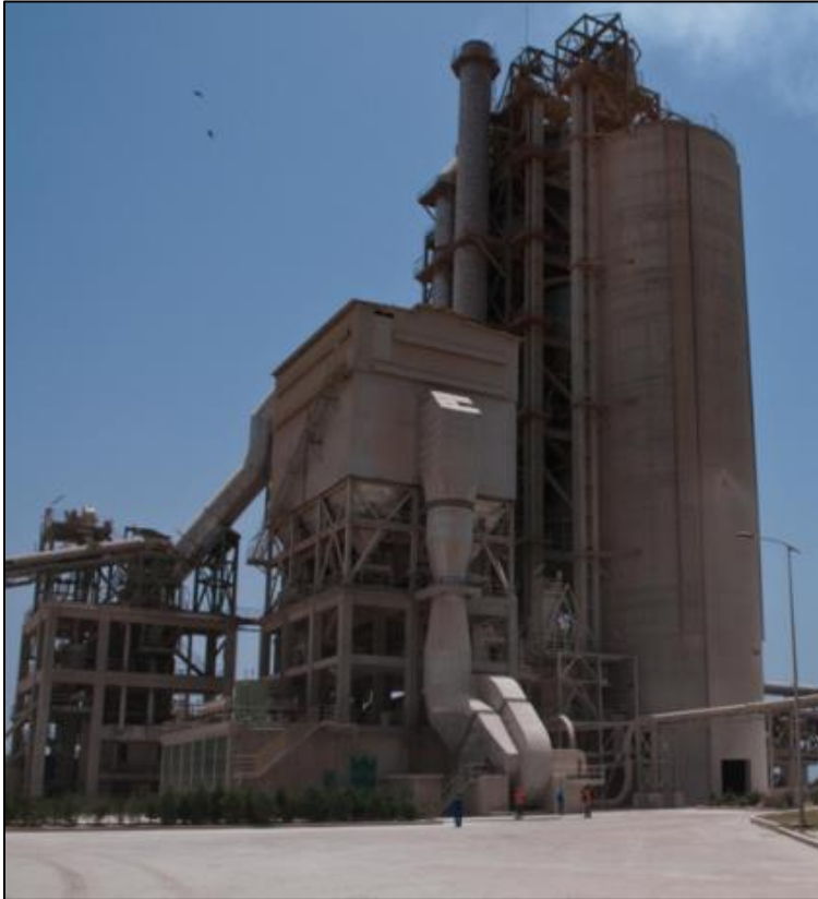
Cement industry in Dakar, Senegal (Credit: Eawag-Sandec)
